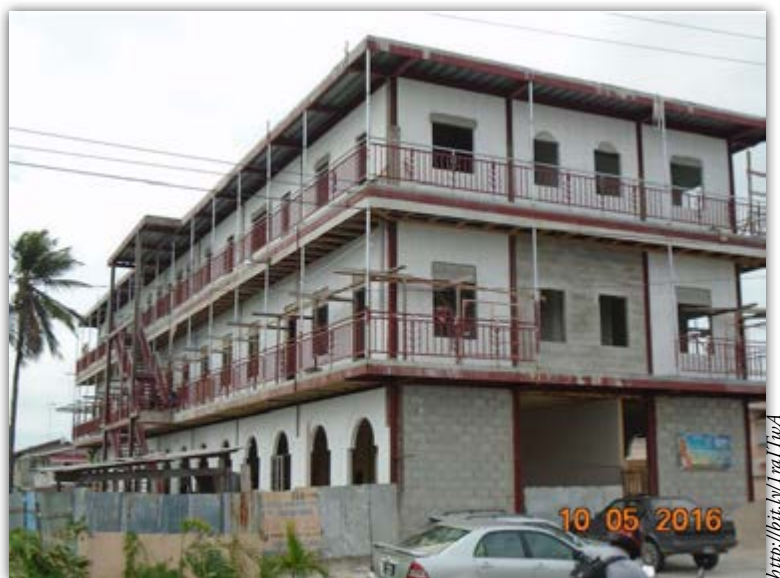
The new temple in Georgetown, under construction
